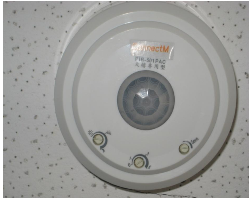
PIR Sensor (Custom Designed)
